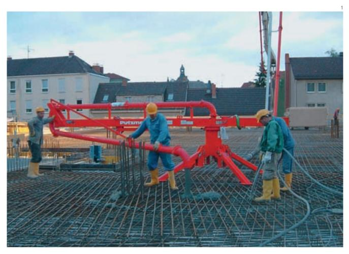
Mechanical distributors lend themselves perfectly where placement using truckmounted pumps and stationary placement booms reach their technical and cost-efficient limits; i.e.
